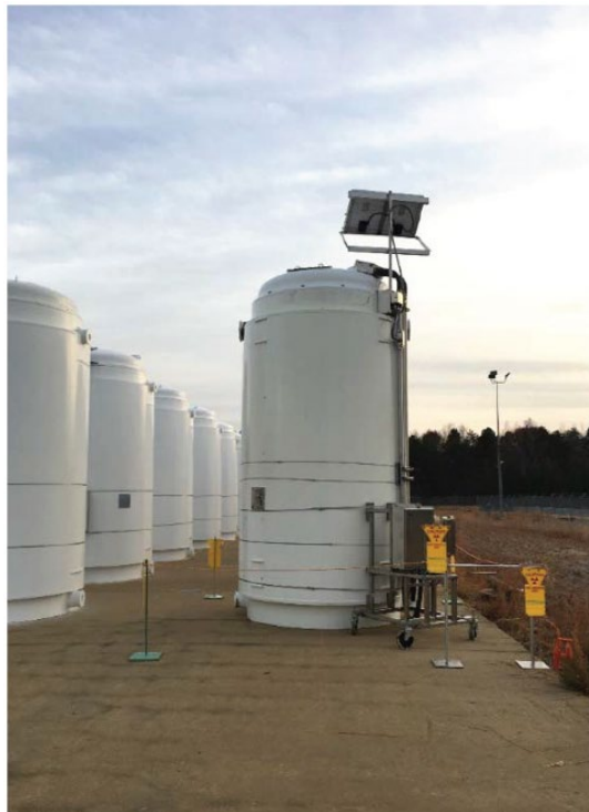
Figure G-1. TN ® -32 cask manufactured by AREVA (now Orano). (Hanson 2016a).
