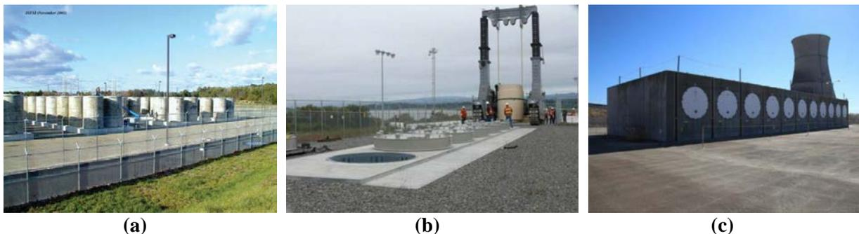
**Figure 3. Types of Dry Cask Storage Systems at Independent Spent Fuel Storage Installations: (a) Vertical, Above Ground (Maine Yankee, Wiscasset, ME), (b) Vertical, Below Ground (Humboldt Bay, Eureka, CA), and (c) Horizontal (Rancho Seco, Herald, CA).** Source: Rechar et al. (2015).
