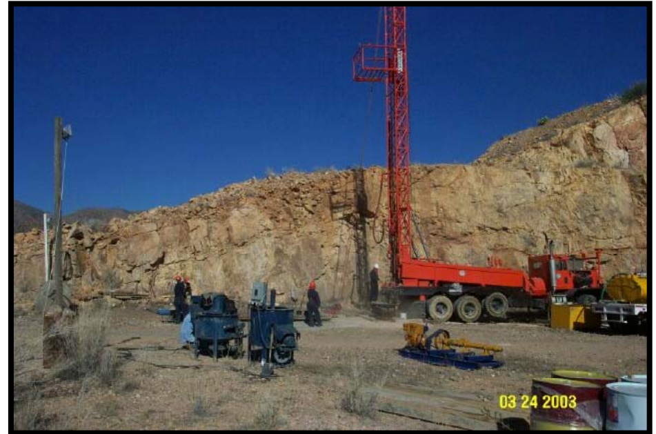
Rig at PB-2 at 30 m
