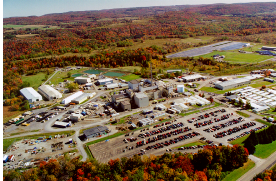
The WVDP is being conducted at a former commercial nuclear fuel reprocessing facility.
