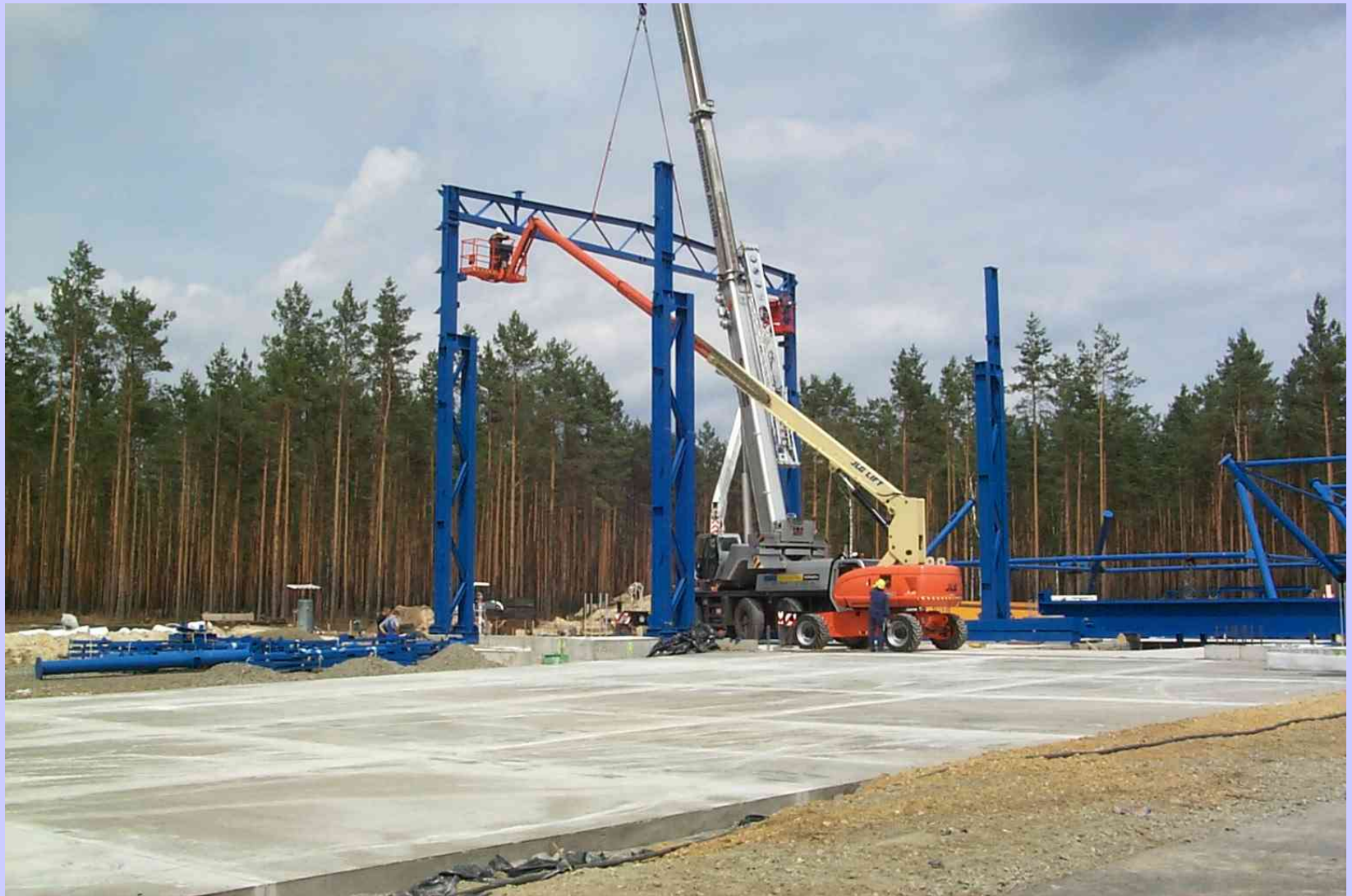
Initial construction work on enclosed test building
