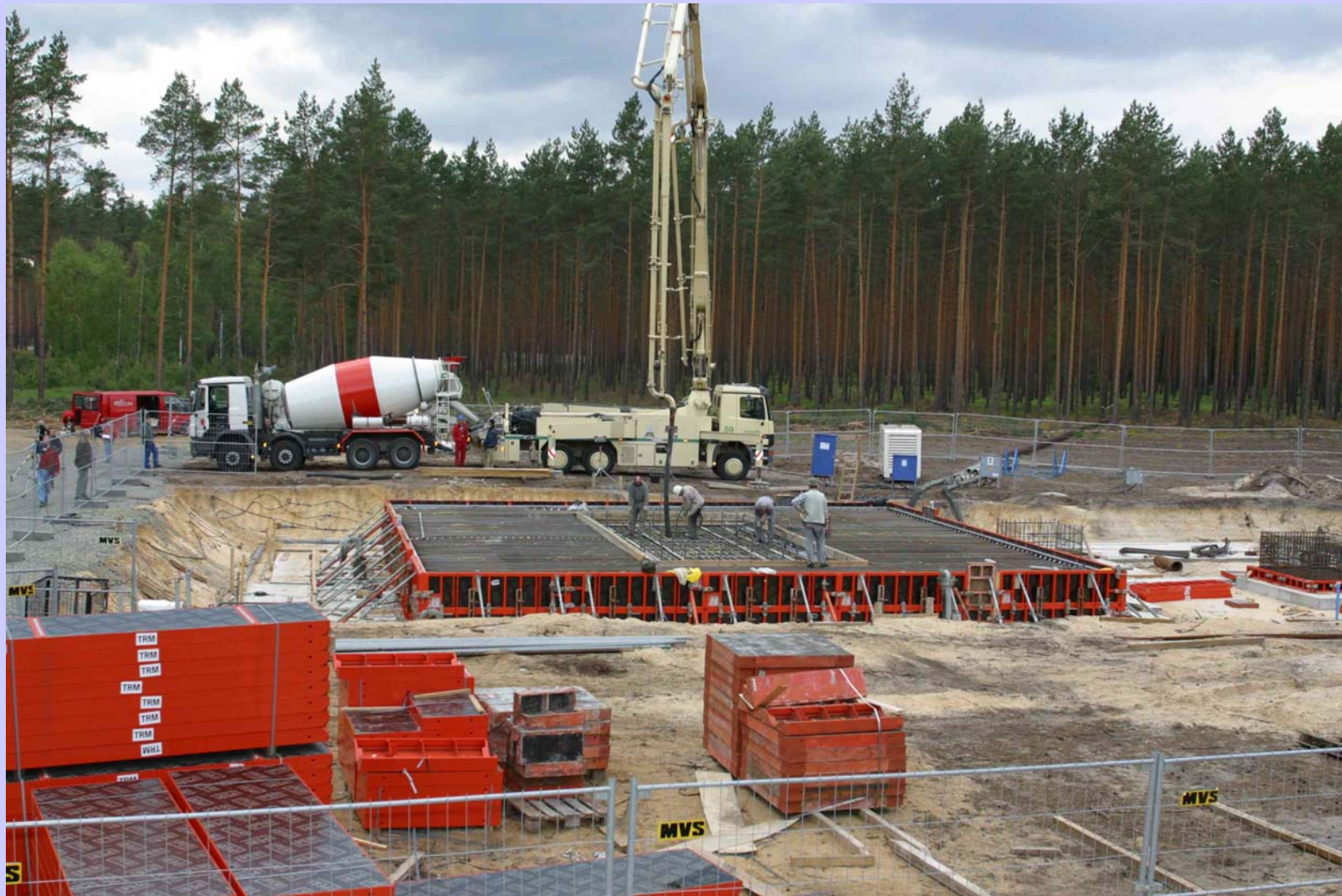
Pouring concrete for the unyielding surface
