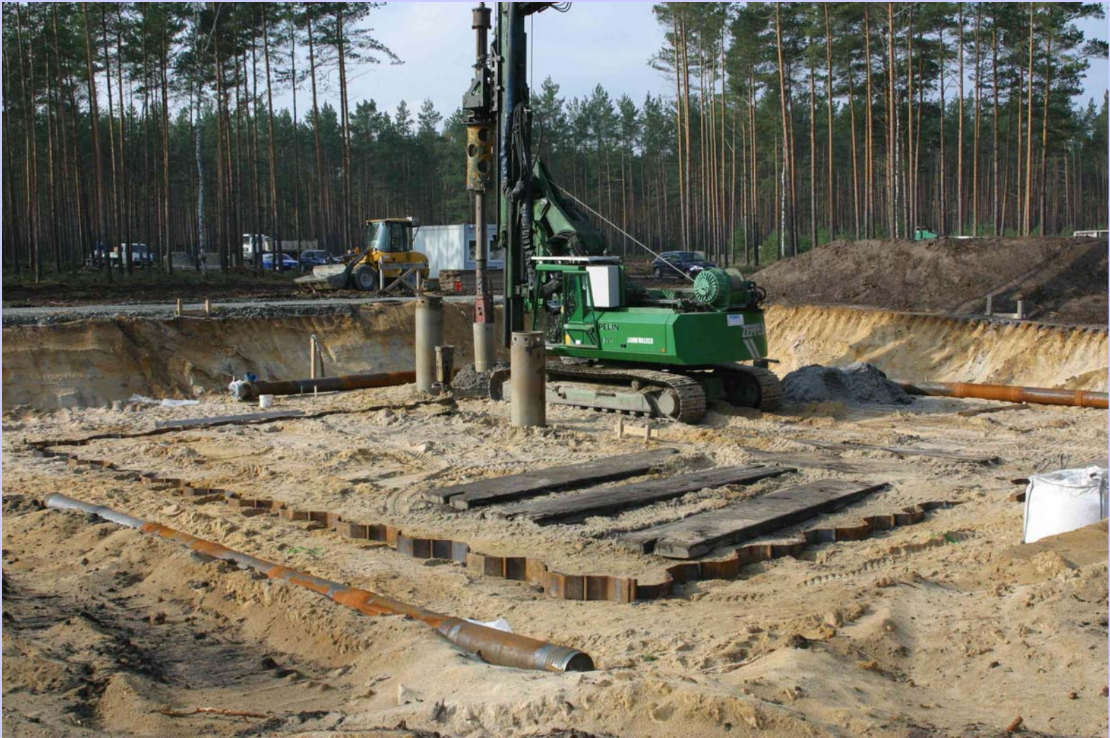
Initial ground excavation and soil preparation
