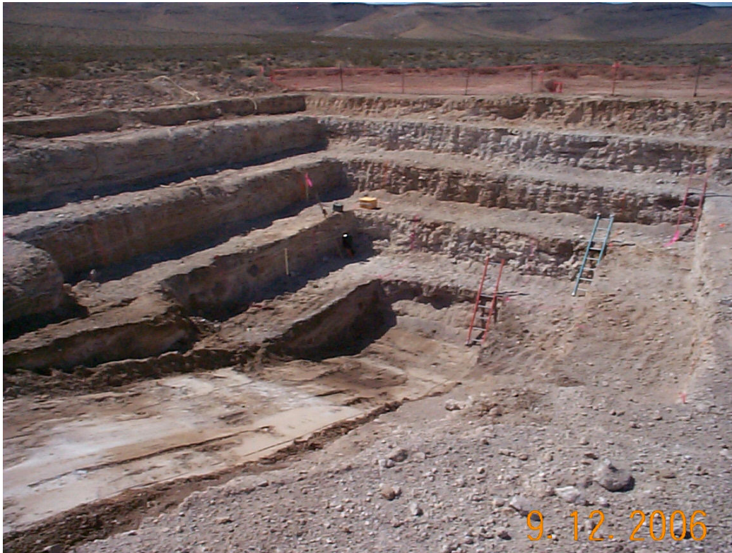
Test Pit in the North Portal Facilities Area
