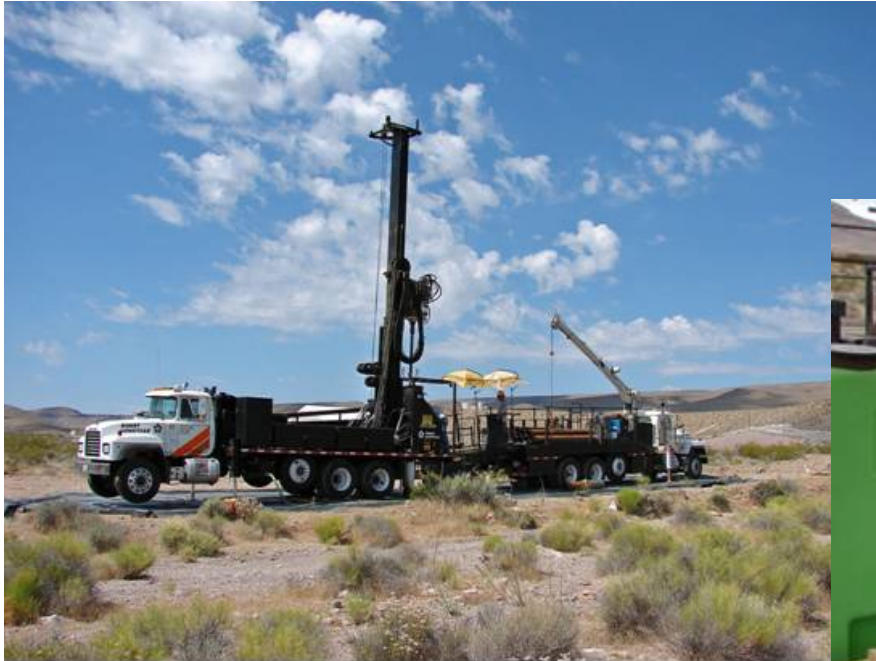
Typical Sonic Core Rig Operation
