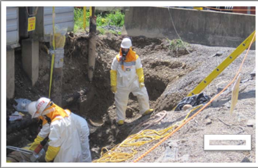
Removal of 16" underground vent pipe header
