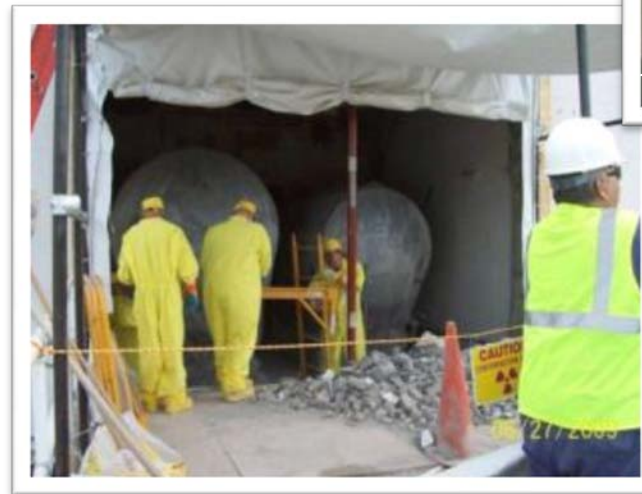
Hot Acid Cell vessel removal
