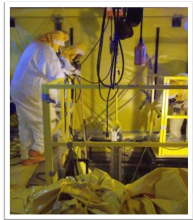
Workers monitor removal of a pump from Tank 8D-4
