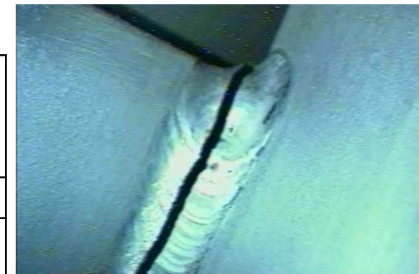
Top weld crack in fuel basket from 15-yr demo at INL
