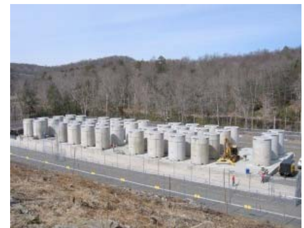
Connecticut Yankee Dry Storage
