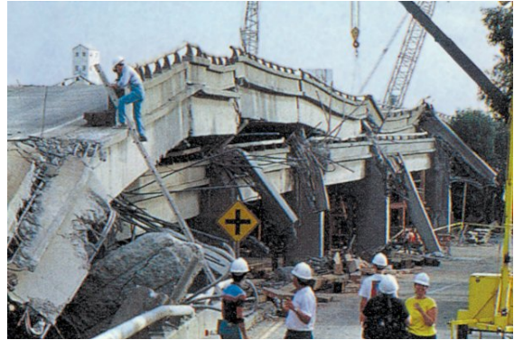
Fig. 3. Cypress Street Viaduct Before and After Collapse
