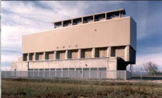
FSV-Vertical modular vault dry storage (Colorado)
