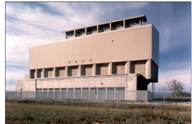
Independent Spent Fuel Storage Installation
