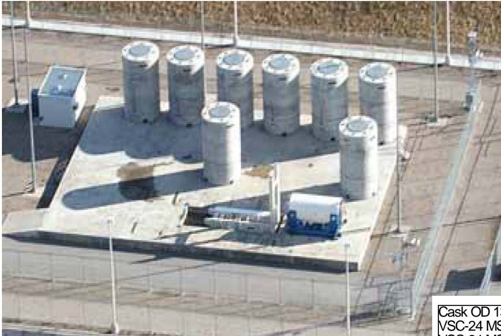
Fuel Solutions System at Big Rock Point
