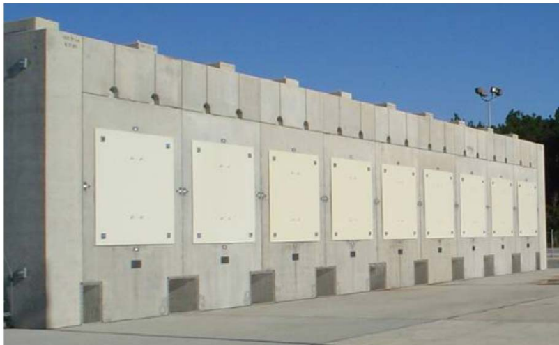
AREVA Transnuclear NUHOMS Storage System at the ISFSI
