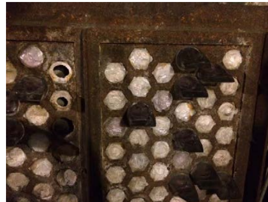
Skylights in Seattle
