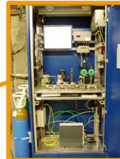
Monitoring of Gas composition within the disposal cell
