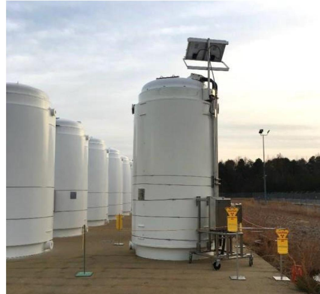
Loaded TN-32B for the High Burnup Demo at North Anna NPP. The solar panel is powering the 63 thermocouples inside the canister. Photo Credit: North Anna NPP
