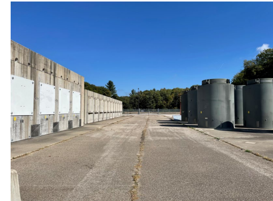
Palisades ISFSI, October 2022
