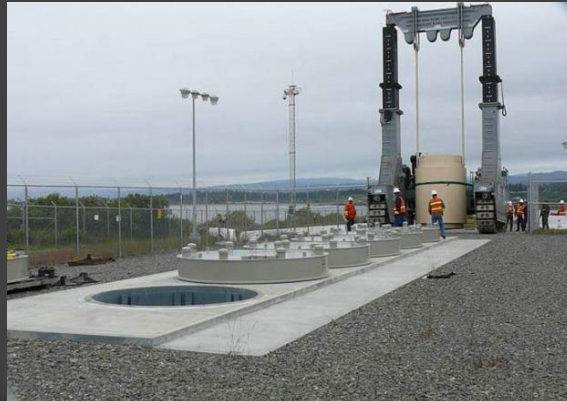
Photo courtesy of Humboldt Bay
