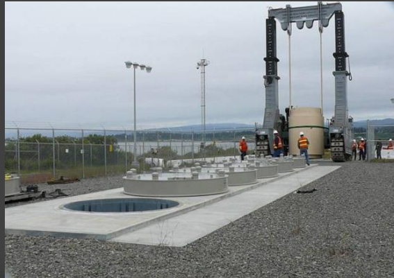
Photo courtesy of Humboldt Bay
