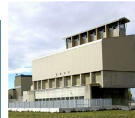
Ft. St. Vrain (CO) SNF Storage
