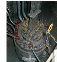
Existing ED installed in H-Canyon
