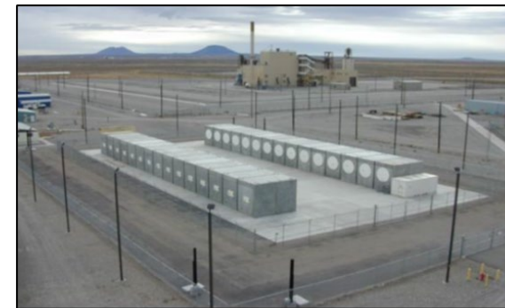
TMI-2 Independent Spent Fuel Storage Facility
