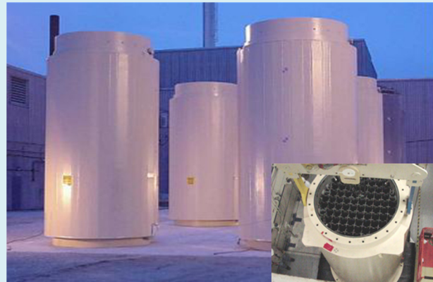
Figure 3-2. Holtec Hi-Star 100 dry storage systems each containing a dual-purpose canister (see inset photo). (Source: Holtec International)
