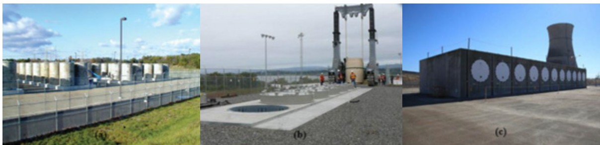
Figure A - 6. Spent nuclear fuel canisters stored in (a) vertical, above ground dry-storage casks, (b) vertical, below ground dry-storage casks, and (c) horizontal storage modules (Rechard et al. 2015).
