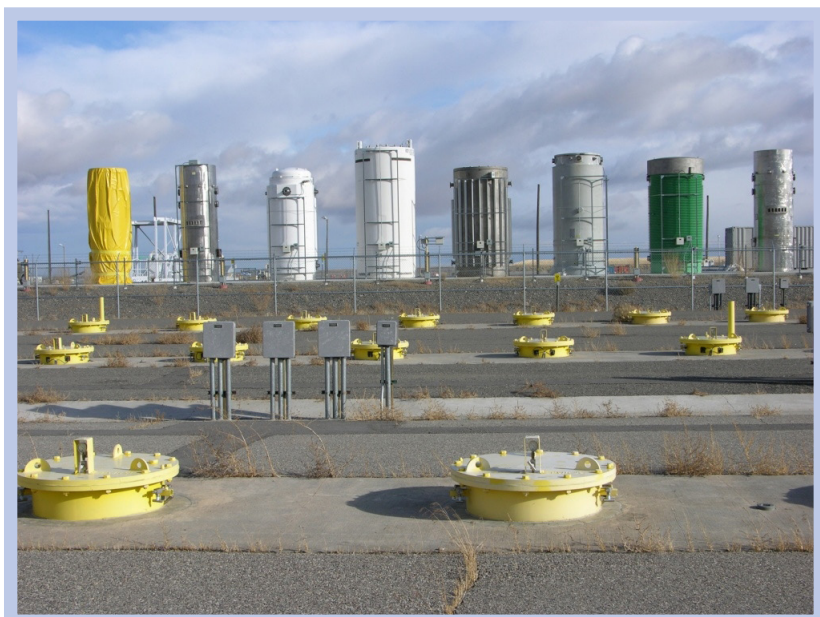
Figure 6. Spent nuclear fuel storage casks at Idaho National Laboratory.
