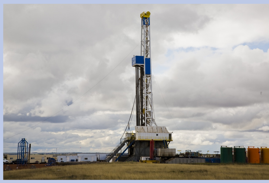
Figure 5. Drill rig for creating deep boreholes.
