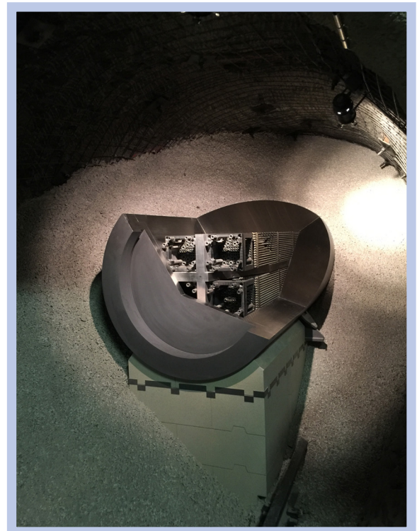
Figure 2. Disposal of spent nuclear fuel in a clay formation.
